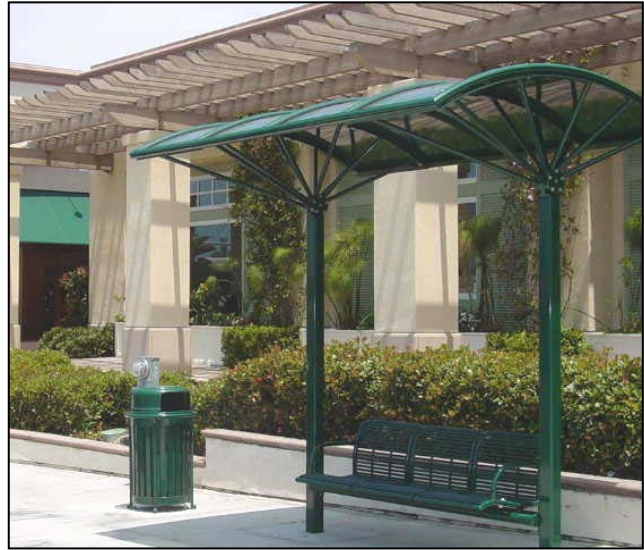
Photo 14: Typical shelter and trash receptacle layout.
