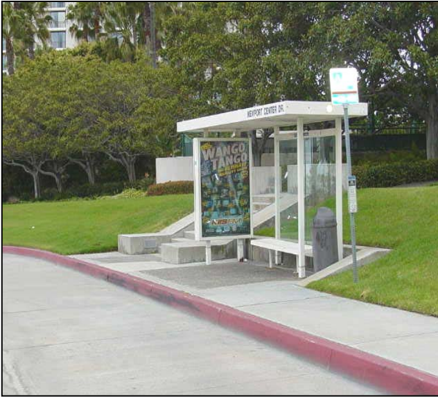
Photo 13: Typical shelter design on narrow sidewalk.
