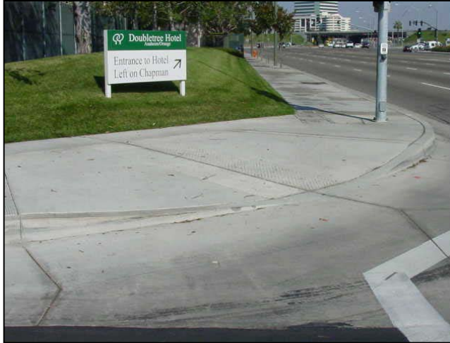
Photo 3: Typical intersection curb ramp.
